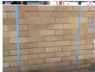
**Allow each test patch to cure for a minimum of 10 days.** Apply paint to the test areas and allow it to cure for at least 48 hours. Using a clean spray bottle, saturate the painted surface with **PHASE II Cleaner** and allow it to dwell for 5 minutes. Re-saturate the surface with **PHASE II**, agitate with a nylon bristle brush and rinse with water. Evaluate the aesthetics and ease of graffiti removal from each test patch to select the most appropriate product combination.
