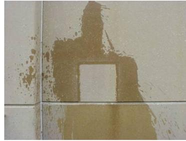
Fig 2. Water sprayed on wall shows the 2'X2' area does not absorb any water
